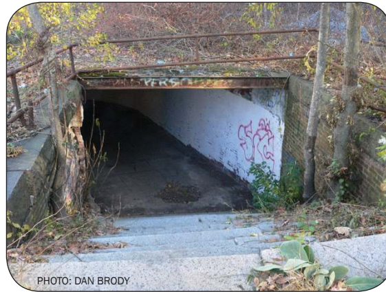
PHOTO: DAN BRODY Pedestrian Underpass Below the Commuter Rail
