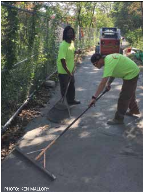
City workers apply a new surface of crushed stone along the so-called “spur” that leads to Needham Street.
