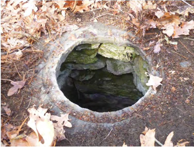
Figure 31. Stone cesspool west of toolhouse.
