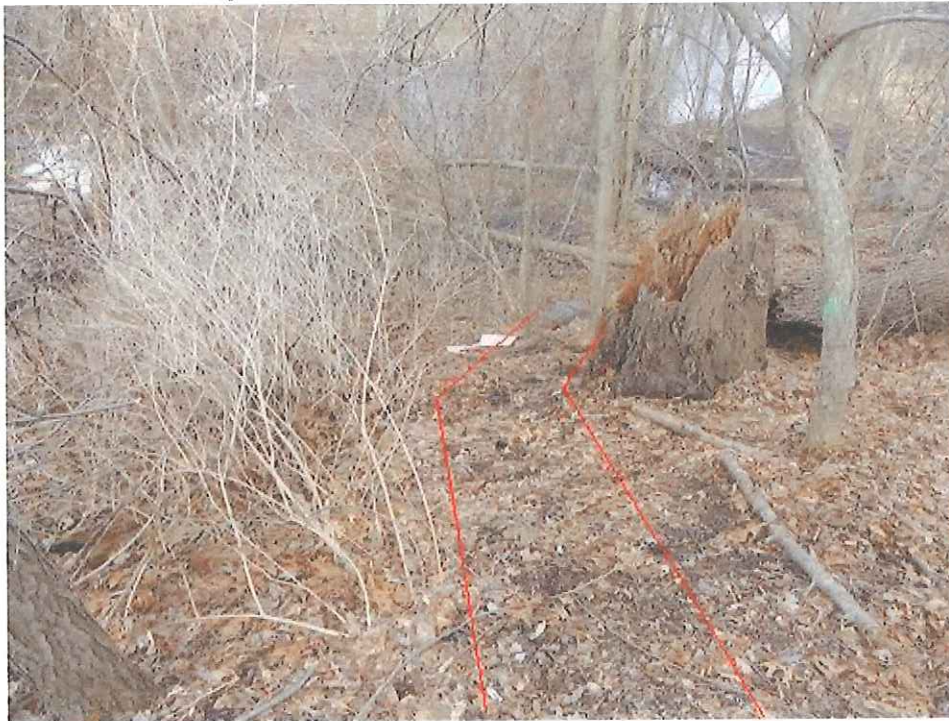
Picture of trail as you head down on the path from the road, steep slope requiring steps and retaining wall:
