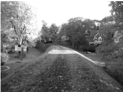
View of aqueduct trail through a residential area of Newton. (Photo courtesy of Newton Conservators Website)
