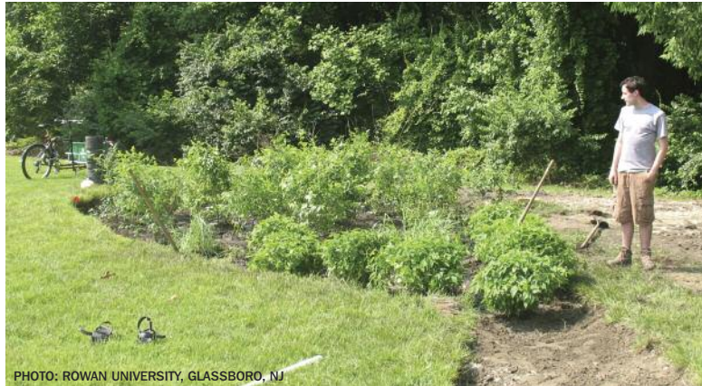
A rain garden has a bowl shape to collect the rain that runs off from a roof, driveway, parking area or yard.
