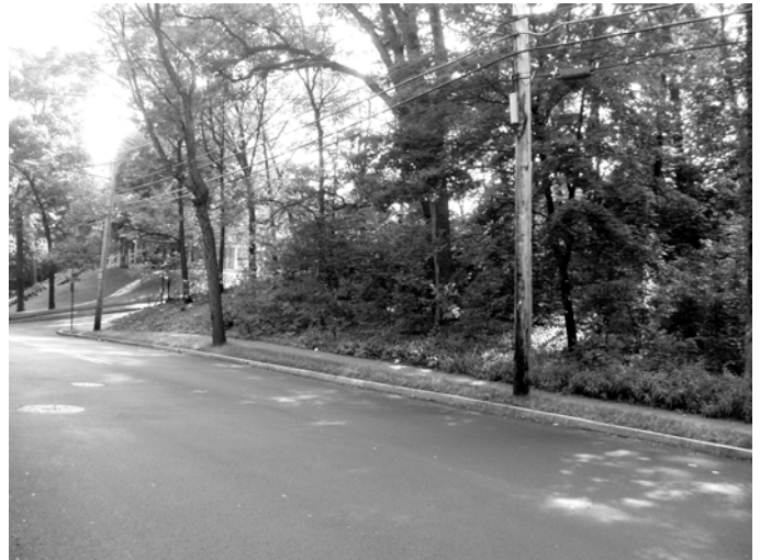
New curbing installed along Grant Avenue at Ordway Park.
