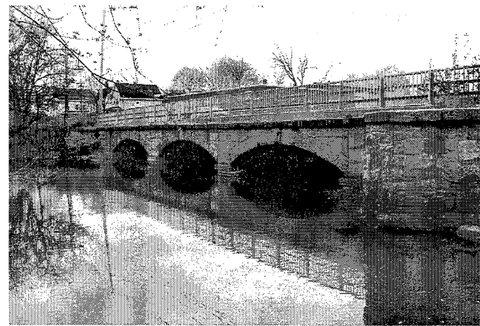
Newton Street Bridge
