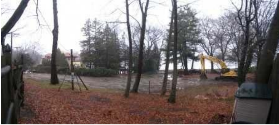
Hannon Property (after demolition) with 230 Lake Ave in background
