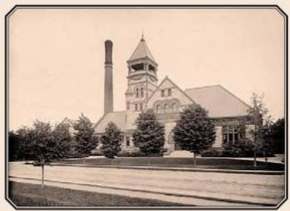
The Chestnut Hill Pumping Station circa 1868 Photo courtesy of Metropolitan Waterworks Museum
