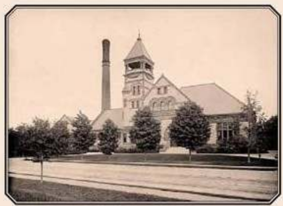
The Chestnut Hill Pumping Station circa 1868 Photo courtesy of Metropolitan Waterworks Museum
