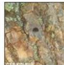
D-shaped Exit Hole
