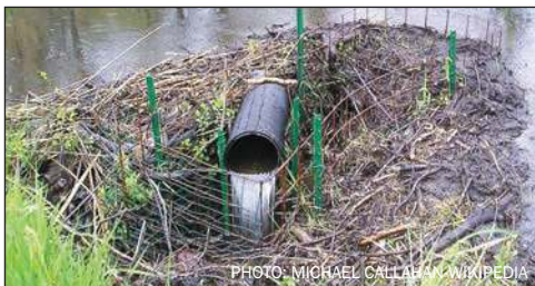
Waterflow control device. The culvert fence and pond leveler pipe is still working after beavers attempt to rebuild dam in 2004.
