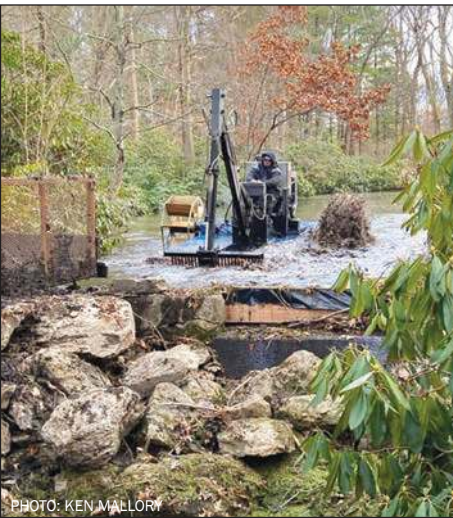
Hydroraker near dam
