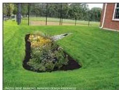
PHOTO: BOB LANGRISH, LANDSCAPE DESIGN PHOTOGRAPHY Oak Hill Middle School roof runoff is piped to the rain garden, where the water slowly seeps into the ground. During large storm events, overflow is directed to the domed open grass.
