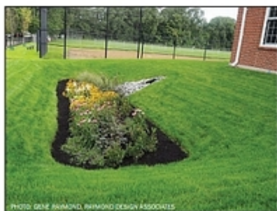
PHOTO: GENE HARMOND, HARMOND DESIGN ASSOCIATES Oak Hill Middle School roof runoff is piped to the rain garden, where the water slowly seeps into the ground. During large storm events, overflow is directed to the domed open grate.
