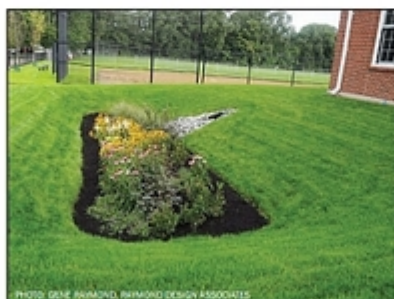
PHOTO: GENE HARMOND, HARMOND DESIGN ASSOCIATES Oak Hill Middle School roof runoff is piped to the rain garden, where the water slowly seeps into the ground. During large storm events, overflow is directed to the domed open grate.
