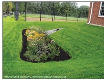
PHOTO: GENE FARWELL, FARWELL DESIGN ASSOCIATES Oak Hill Middle School roof runoff is piped to the rain garden, where the water slowly seeps into the ground. During large storm events, overflow is directed to the domed open gate.
