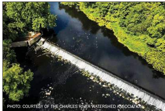
Aerial photo of the Watertown Dam
