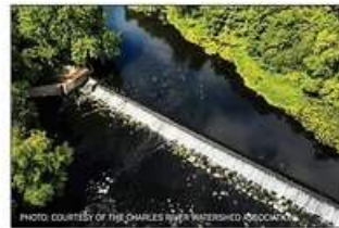
Aerial photo of the Watertown Dam
