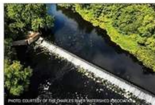
Aerial photo of the Watertown Dam
