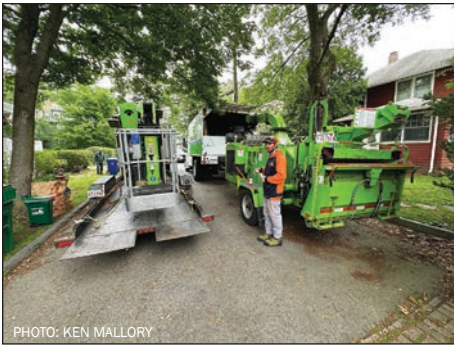
Tree removal from private property in Newton
