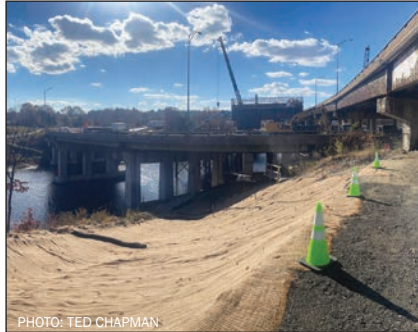
Pigeon Hill I-90 West: Looking west from Pigeon Hill, the new piers for I-90 east roadway are rising across the Charles River 40 feet south of I-90s current location. The Pigeon Hill Trail will run under this roadway.
