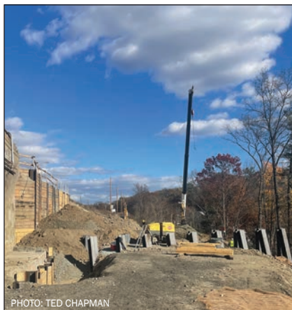
Pigeon Hill I-90 east: Looking east from Pigeon Hill the steel foundation for the abutment under construction; the Pigeon Hill Trail will run downhill on a shelf created to the right (river side) of the new abutment.
