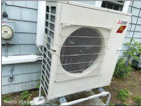
Mini split heat pump used for home heating during winter and cooling during summer.
