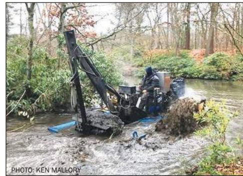
PHOTO: KEN MALLORY Hydro-raking of the pond is part of the needed maintenance.
