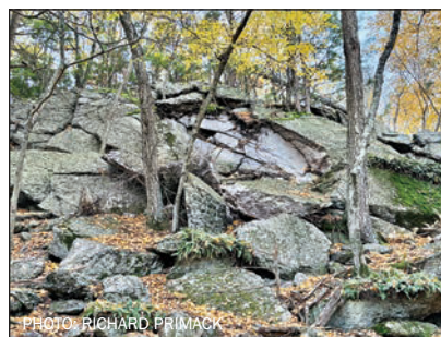
Hemlock Grove (7) with rockfall
